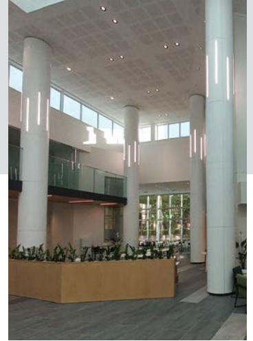
Toyota HQ, Palmerston North - curved aluminium column cladding
