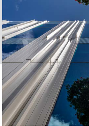
University of Auckland, B201 - unitised aluminium plank
