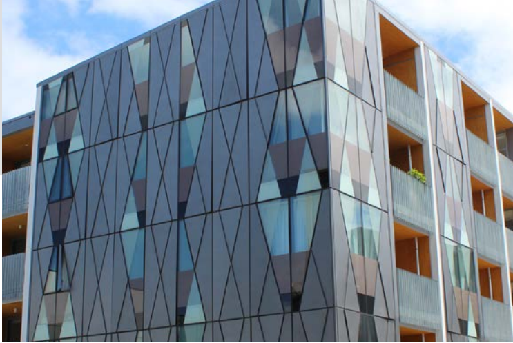
Aria Apartments, Vinegar Lane, Auckland - architectural folded aluminium
