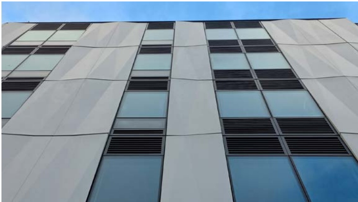
1 Enfield Apartments - architectural aluminium pressings integrated into curtainwall
