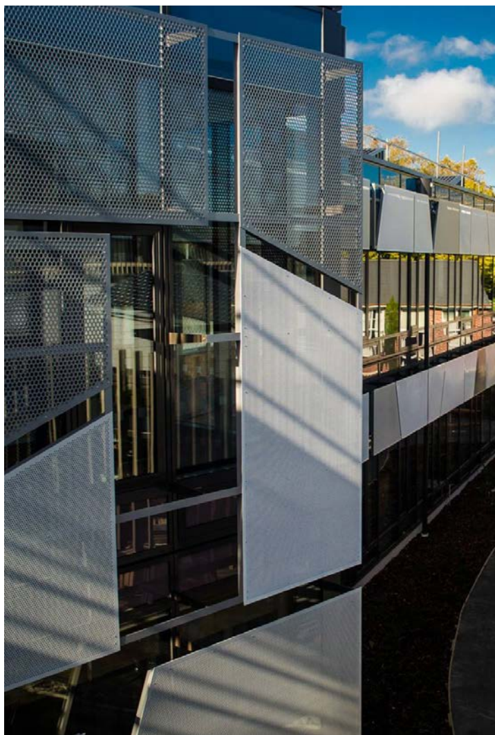
Rangī Ruru Girls School, Christchurch, perforated metal sunscreens to Science and General Academic blocks.
