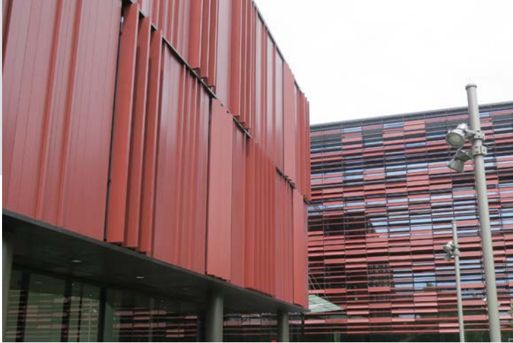
AUT M1 The Mana Hauora Building - facade planking (left), and horizontal solar shading cantilevered off unitised curtainwall
