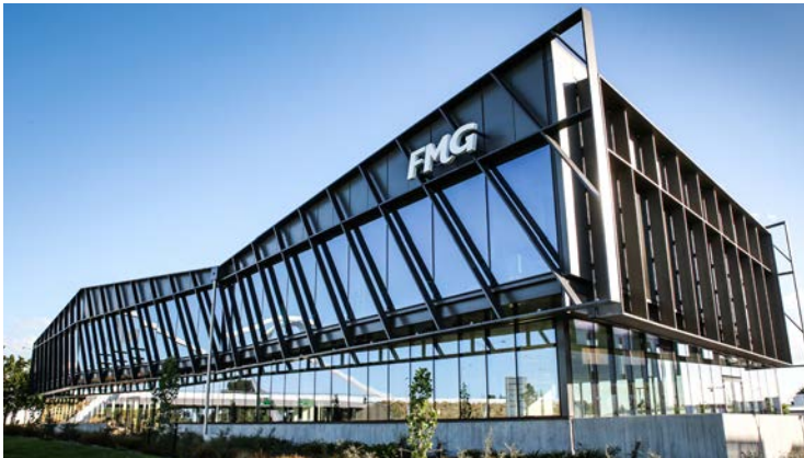
FMG Building - Christchurch - horizontal & diagonal fins with a complex T-section steel bracketry system to connect fins into curtainwall
