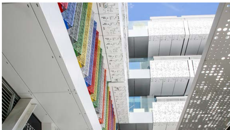
Bnz Cashel stage 2, Christchurch - perforated decorative sheet metal canopies and solar shading
