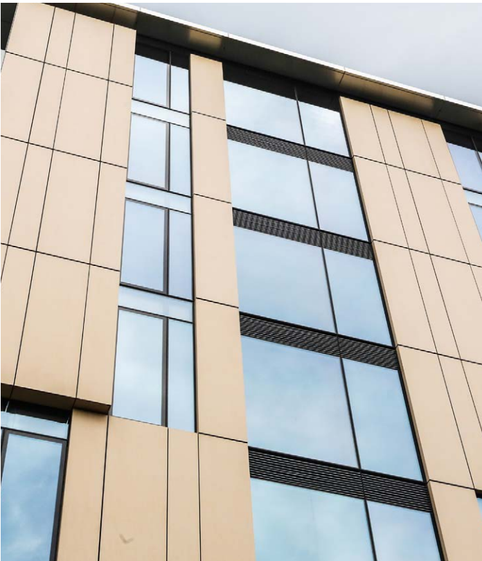
Armagh Apartments, Christchurch - PW100 suite integrated with large format porcelain panels.
