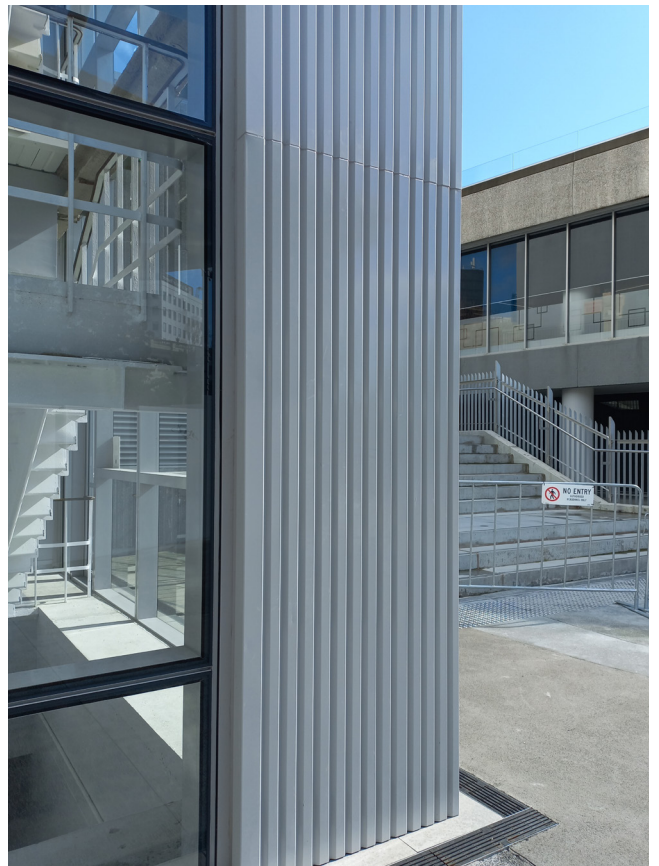
CAB Apartments, Auckland - unique folded metal cladding designed to match the original heritage fluting.
