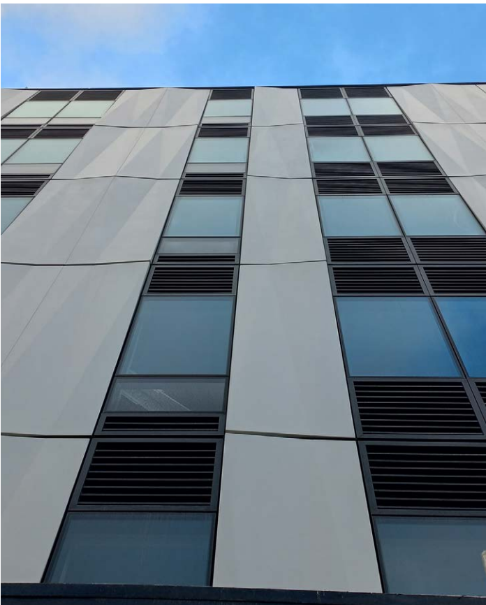
1 Enfield Street Apartments, Auckland - PW1000 integrated with architectural aluminium feature pressings
