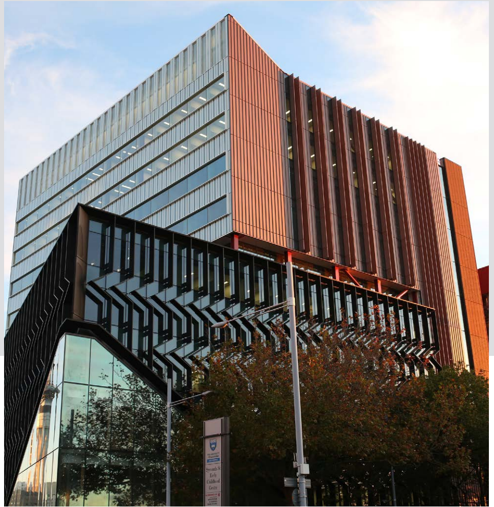
UOA School of Science 302 - PW1000 unitised curtainwall integrated with aluminium feature chevrons to upper podium, and incorporating glazed and Zinc clad integrated panels and Zinc clad feature fin projections to upper tower.
