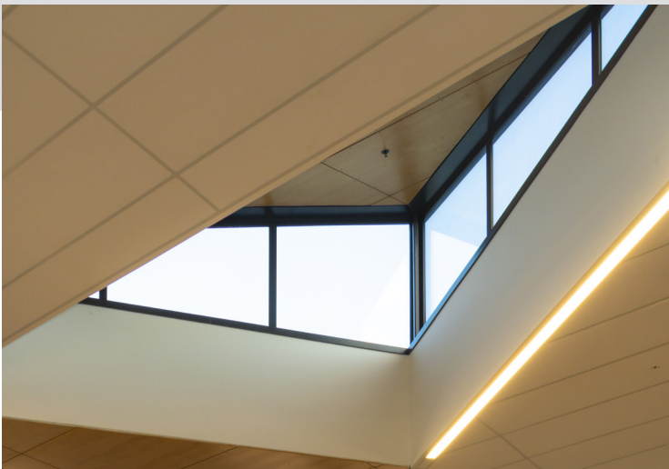
Waitohi Johnsonville Library, Wellington - Delta Suite celestery windows
