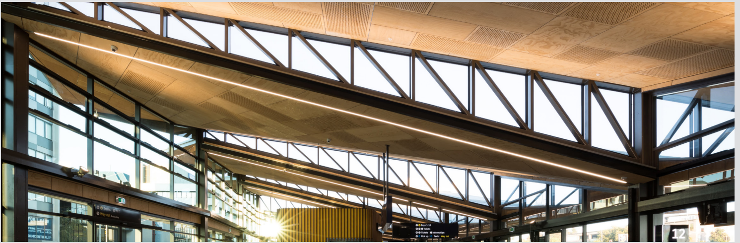
Manukau Bus Interchange, Auckland - Delta Suite sawtooth rooflights
