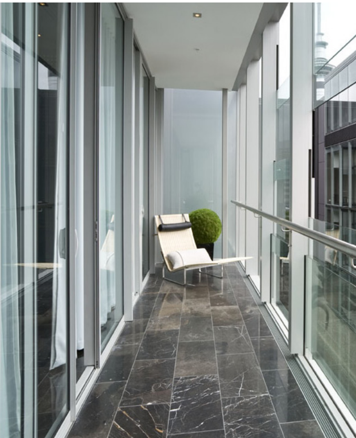
Stamford Plaza Apartments, Auckland - Twin Skin Facade with Thermosash PW1000 outer skin and Delta Suite acoustic sliders to the inner skin.
