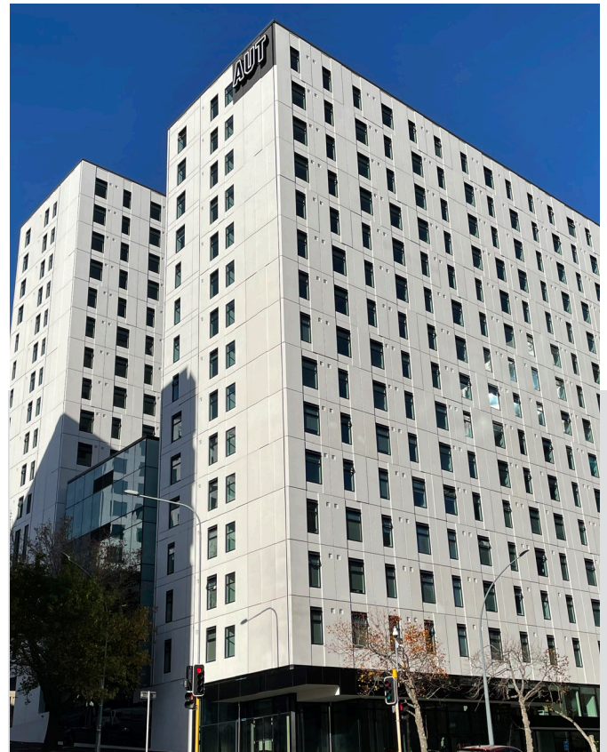
AUT Student Accommodation DELTA SUITE WINDOWS
