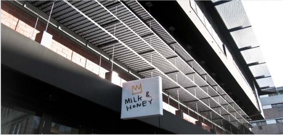
Shadetread™ installed to facade as external trafficable sunscreens - Victoria University, The Hub, Kelburn Campus
