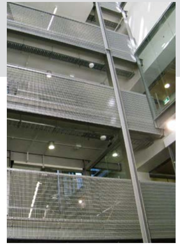
Shadetread™ externally integrated in PW1000 flush glazed curtainwall and Shadegrade™ as internal balustrades - Telecom Tower, Willis St, Wellington
