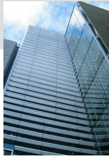
Shadetread™ externally integrated in PW1000 flush glazed curtainwall and Shadegrade™ as internal balustrades - Telecom Tower, Willis St, Wellington
