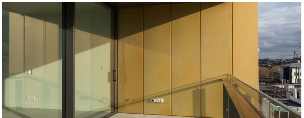
Halsey St, Auckland - RS1000 Cladding System
