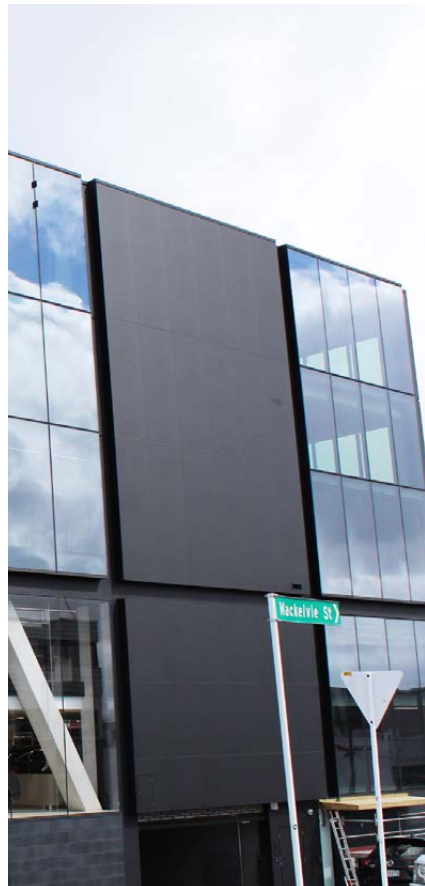
Giltrap Prestige Building, Auckland - WS1000
