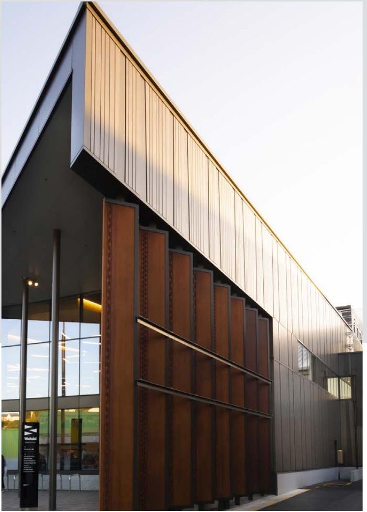
Johnsonville Library - RS1000 Cladding System incorporating powdercoated aluminium vertically and horizontally fixed
