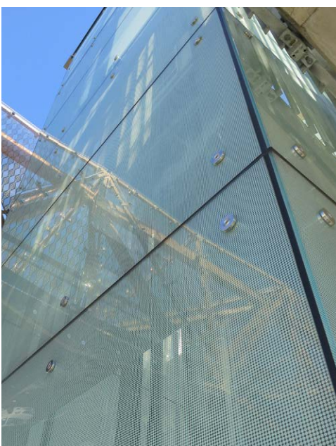
Jacobs ladder lift shaft, Auckland - structurally glazed with patch fittings.
