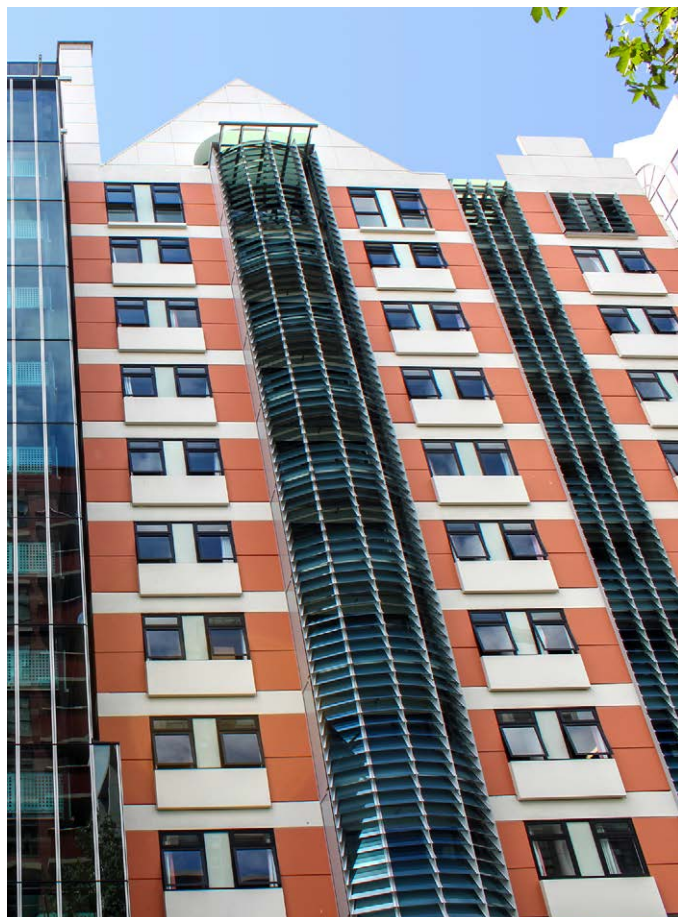
University of Auckland, O'Rorke Hall - glazed louvres integrated with aluminium rainscreen.
