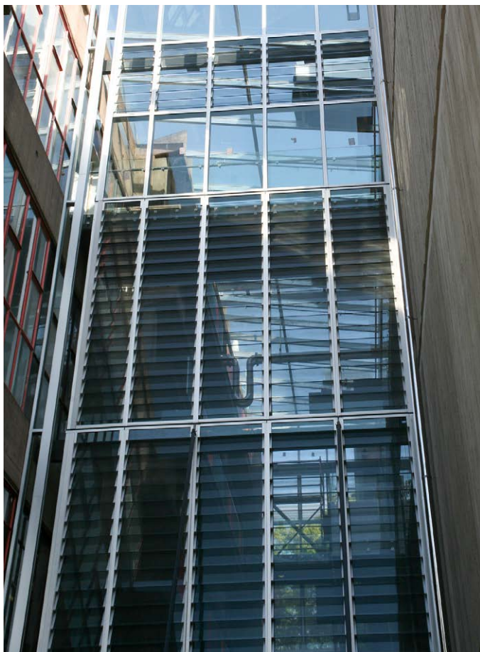
University of Auckland, Thomas Building - structural glass louvres
