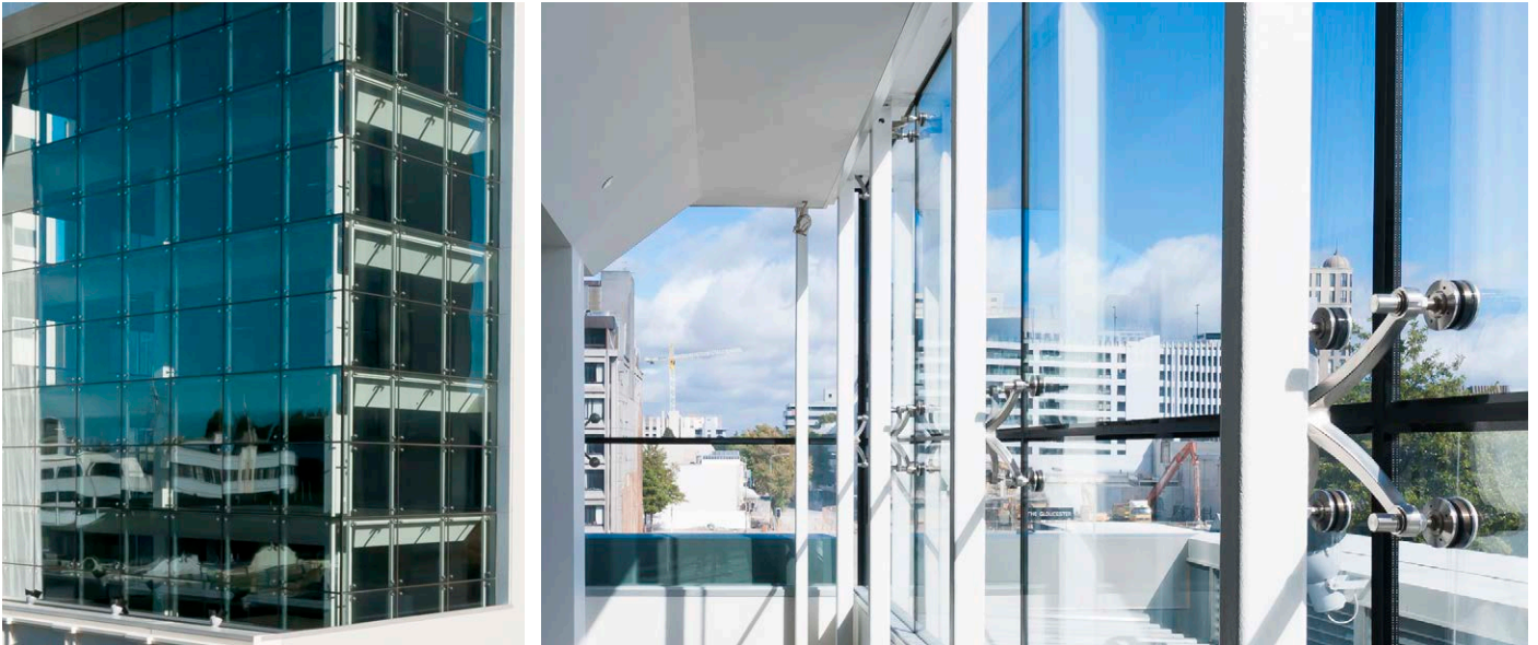
The Press Building, Wellington - completed prior to the 2021 earthquake features a double glazed spider fixed facade.
