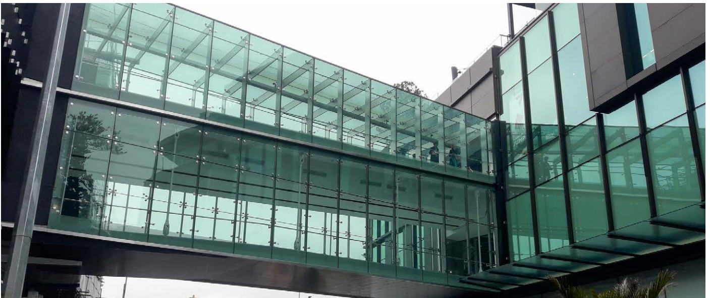
Westfield Newmarket, Auckland - structurally glazed pedestrian bridge with spider fittings.
