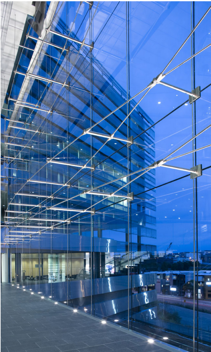
University of Auckland Business School - bow truss structural glass assembly to the main entry suspended from the support structure at the roof level.
