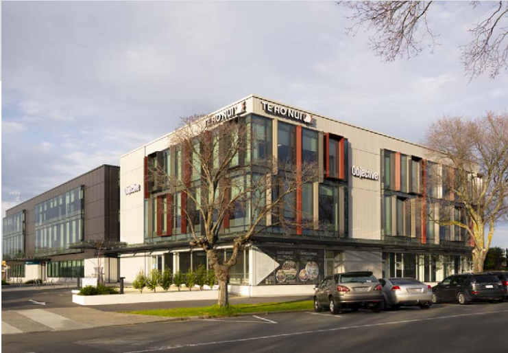
Te Ao Nui (IL4) Building in Palmerston North - PW1000 integrated with solar shading, and cladding (plank / folded sheet metal / fixed rainscreen systems)
