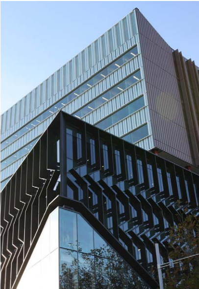
University of Auckland SCIENCE CENTRE (BUILDING 302)
