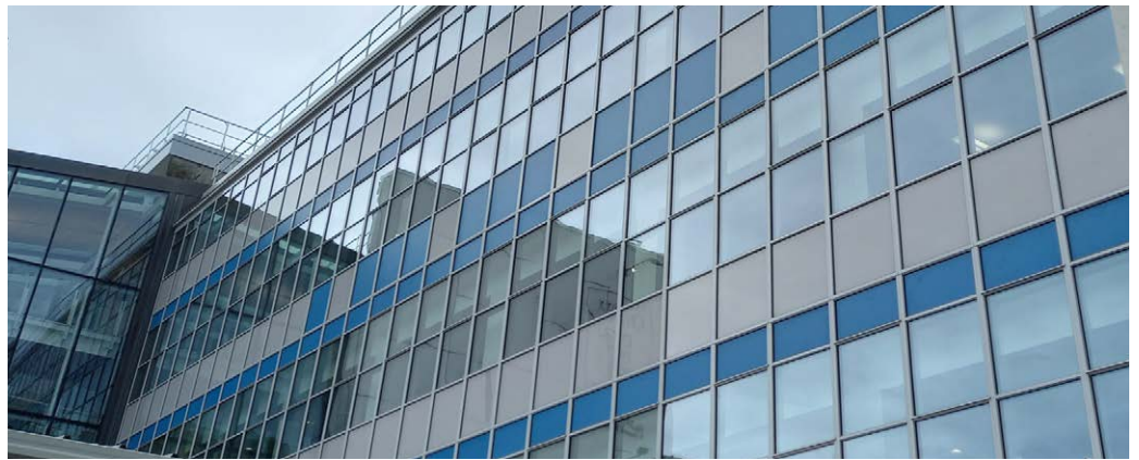
UO Dental School, Walsh Building - PW1000 replicating the pattern and colour of the original 1960s design to maintain the connection to the iconic past facade
