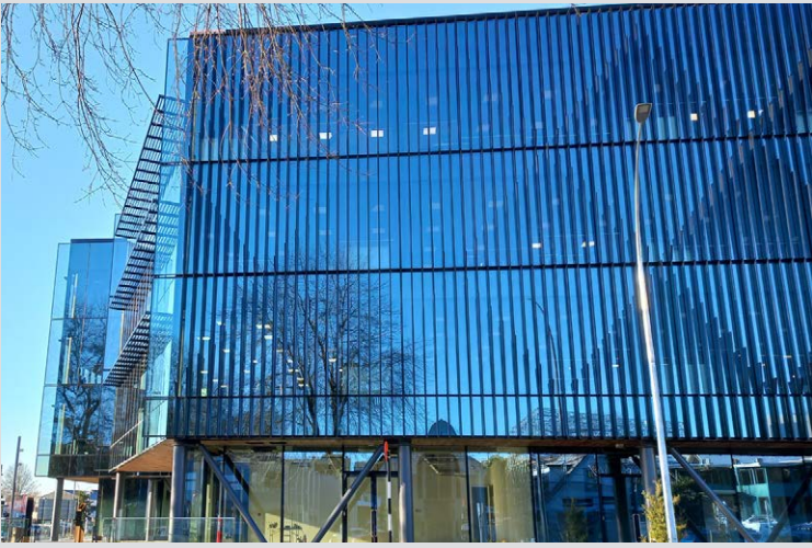
Project Hauata offices for ACC, Hamilton - PW1000 with integrated vertical box louvre fins, and horizontal solar shade louvres.
