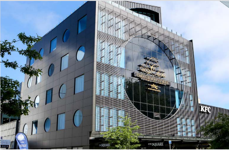
699 Comobo St Hotel, CHCH - PW1000 integrated with a custom solar shade
