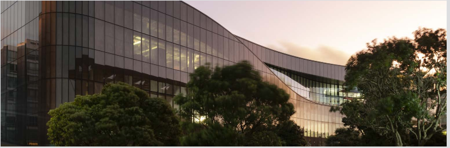
Tākina Wellington Convention and Exhibition Centre is a sustainable 5-Green Star building featuring Thermosash PW1000 Unitised curtainwall comprising of 1000 individual panels made up of 1500 pieces of SEFAR® glass.
