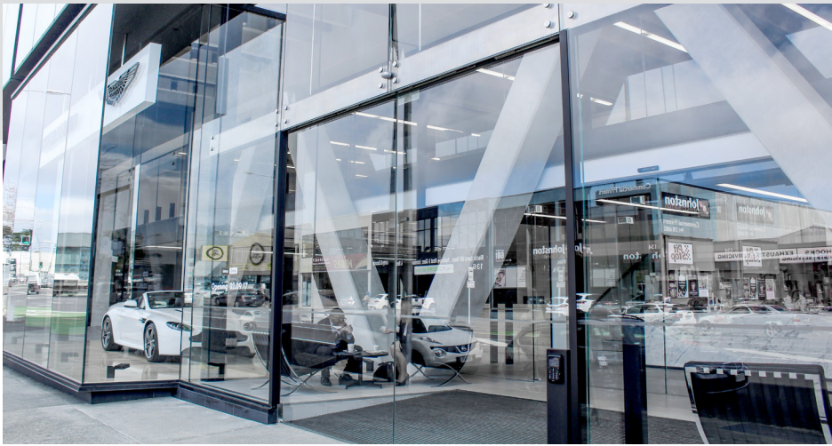
Giltrap Prestige, Auckland - channel glazed showroom with integrated glass fins and framed glass auto doors
