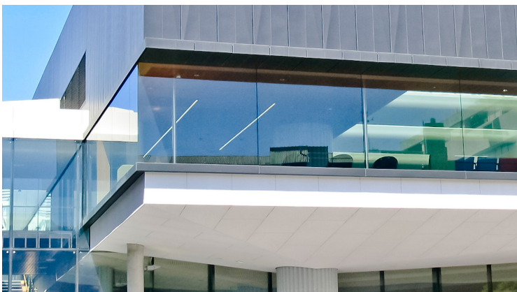
Victoria University Wellington, The Hub, Kelburn Campus - channel glazing to upper level
