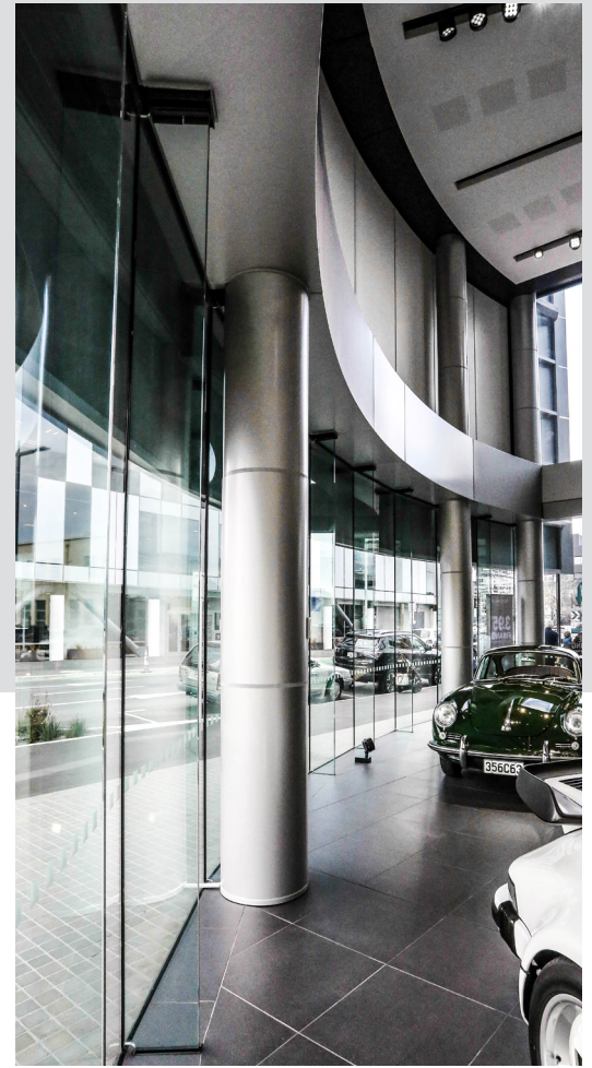
Medcar Porsche, Christchurch - showroom with recessed channel glazing and integrated glass fins
