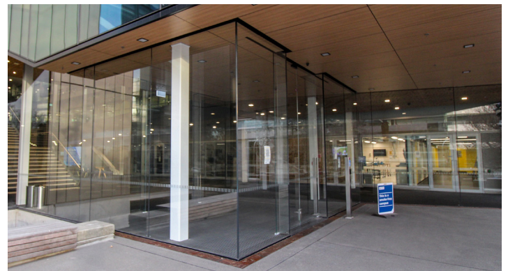
UOA Engineering 405 - channel glazed entrance with frameless glass doors
