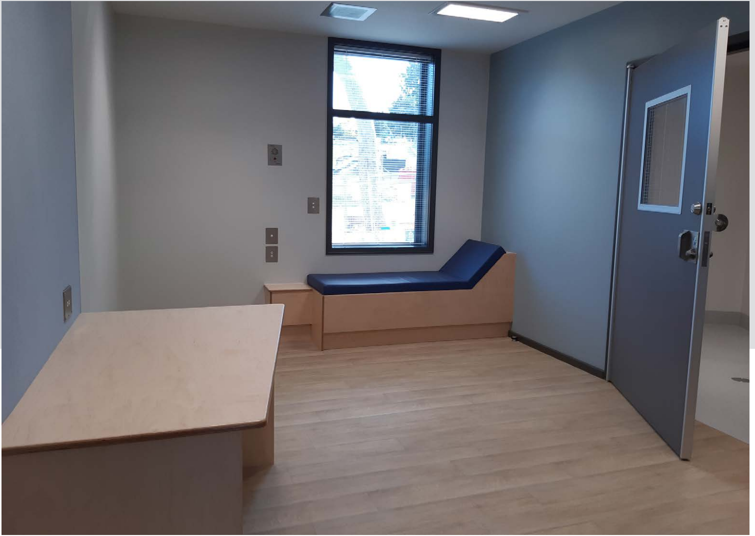
Mason Clinic WDHB - DeltaGuard™ security windows with integrated isolated venetian blinds in rooms
