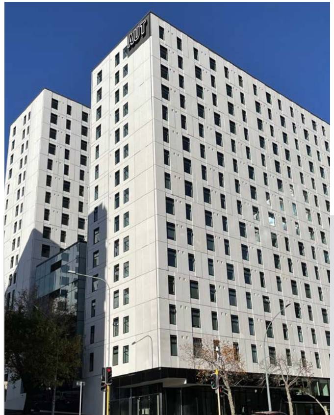
AUT Student Accommodation DELTA SUITE WINDOWS
