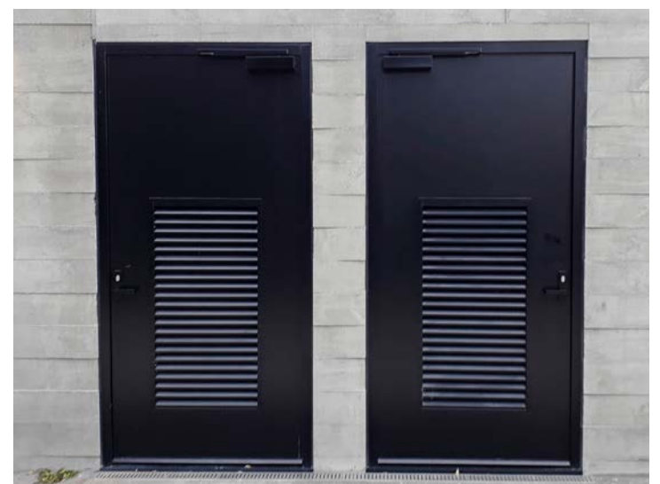
594 - 598 Manukau Rd, mixed use building - Delta doors with louvers
