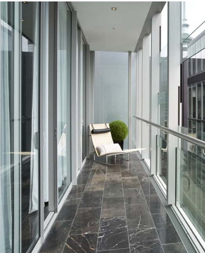
Stamford Plaza Apartments, Auckland - Twin Skin Facade with Thermosash PW1000 outer skin and Delta Suite acoustic sliders to the inner skin.
