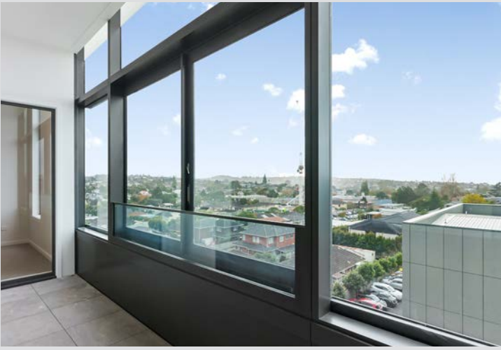
Quest Hotel Takapuna, Auckland - Delta punch windows at Level 4
