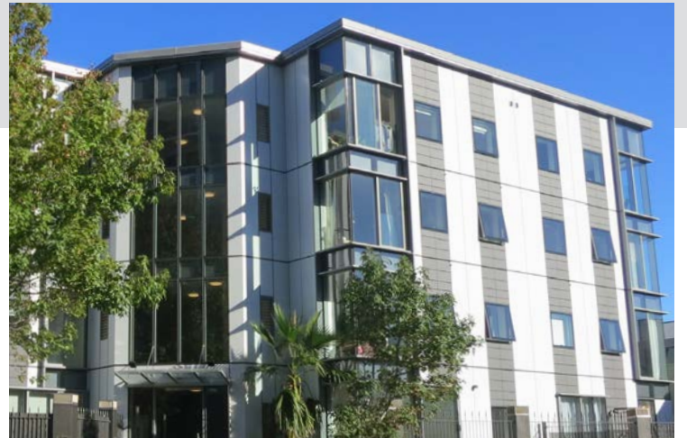
Columbia Apartments, Auckland- Integrated Delta Suite windows & slider balconies
