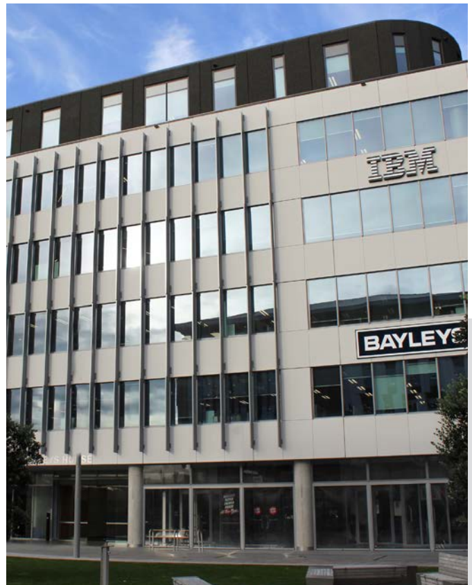
Barclays Building C, Auckland DELTA SUITE FACADE STRIP AND INSERT WINDOWS
