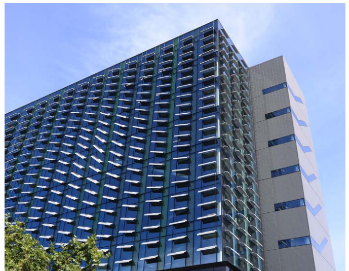
University of Auckland Engineering 405 - fixed external sunshades integrated into Thermosash PW1000 double glazed curtainwall.
