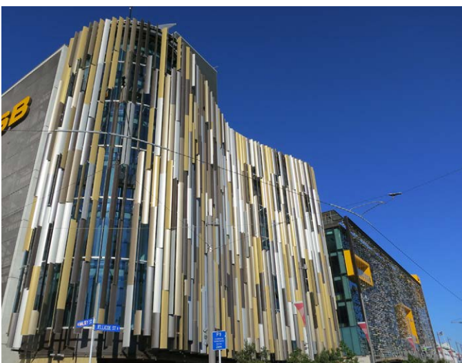
ASB North Wharf, Auckland - vertical solar shade fins suspended off the curtainwall.
