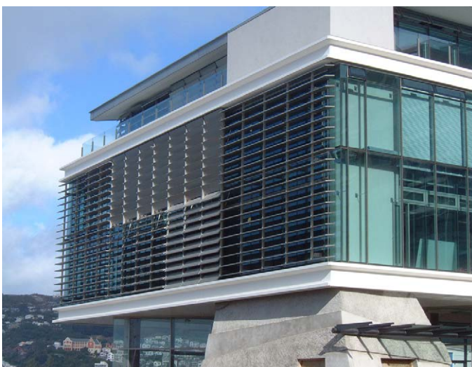
Meridian Energy Site 7, Wellington - automatic window and louvre actuators, providing passive heating and cooling of the building.
