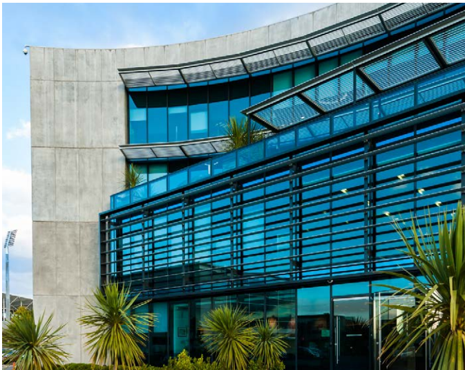
Showplace, Christchurch - PW400 Unitised Curtainwall with integrated horizontal solar shading louvres
