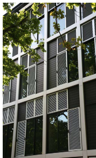
University of Auckland, Thomas Building - integrated sunscreen
