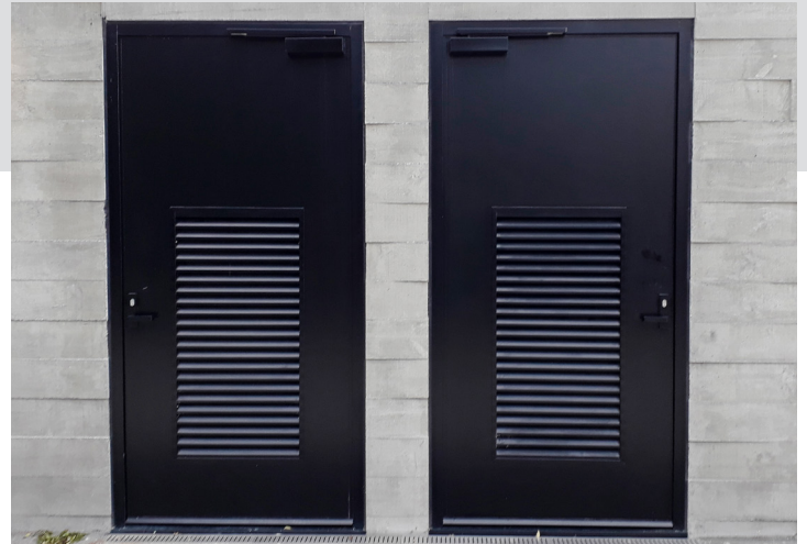
Doors with MAL 40mm Single Bank - 594-598 Manukau Rd, Auckland.
