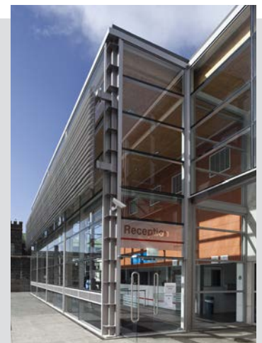
Mt Eden Prison gate house, Auckland - security glass facade
