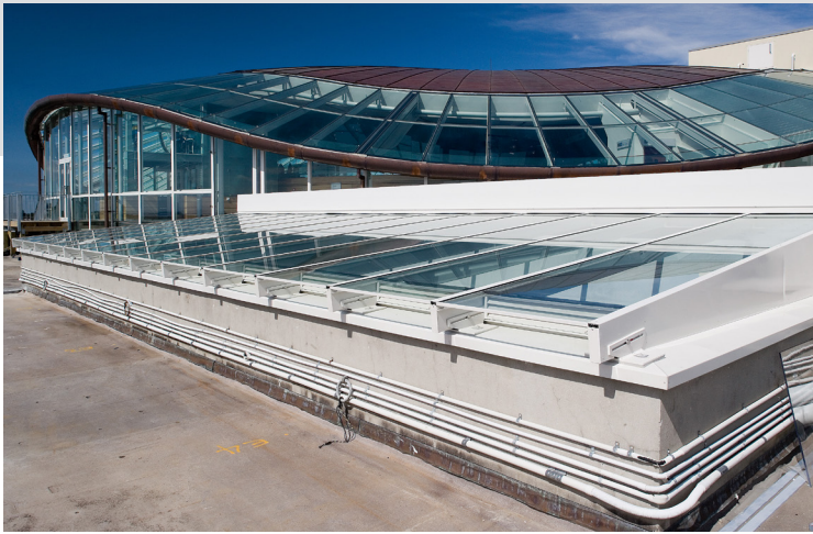
Auckland Museum "The Dome" and rooflights
