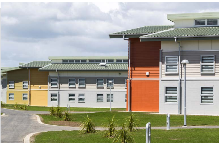
Wiri Prison, Auckland - security windows with bespoke sash.
