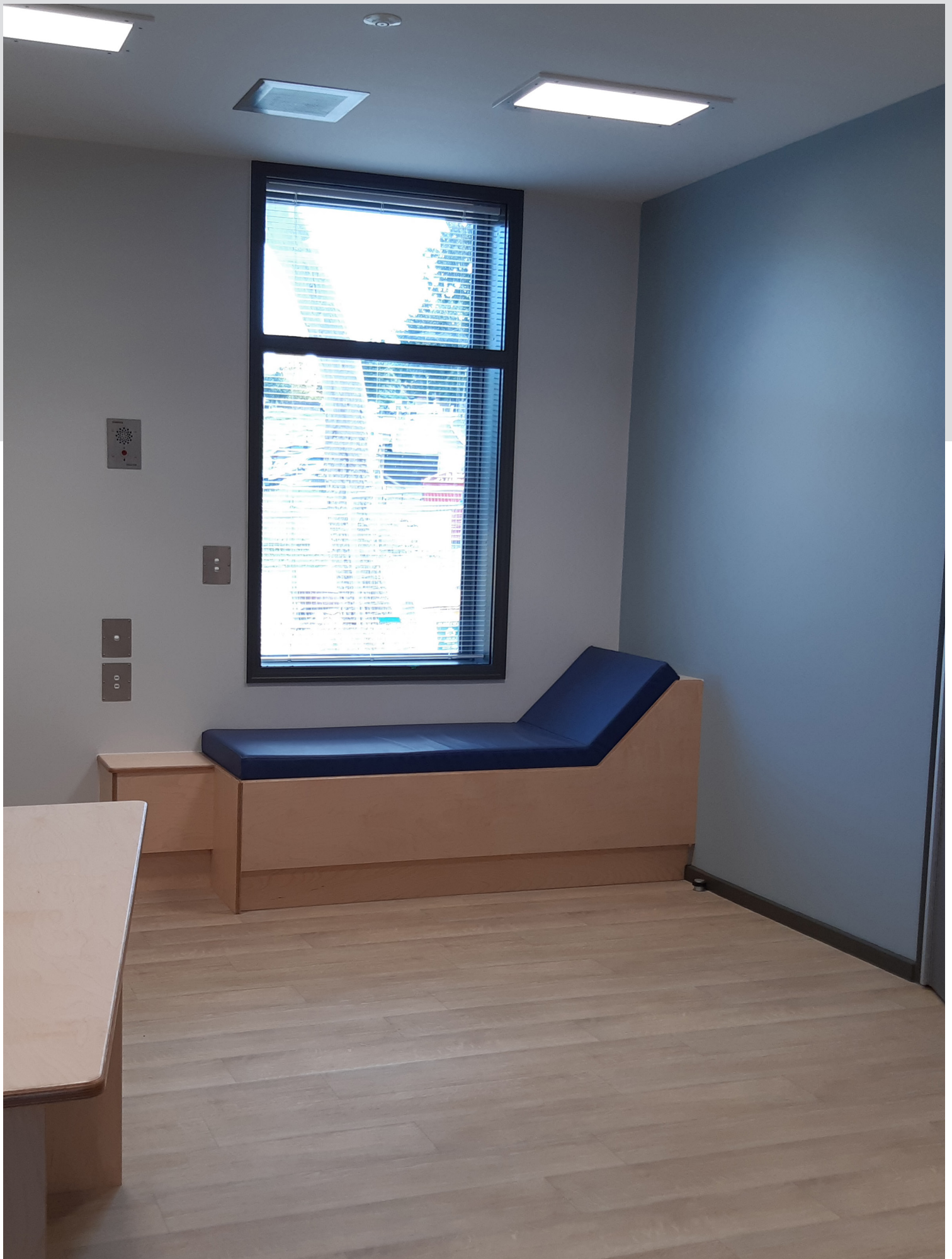
Mason Clinic, Te Whatu Ora, Auckland - DeltaGuard™ security windows with integrated isolated venetian blinds for anti-ligature mitigation.
